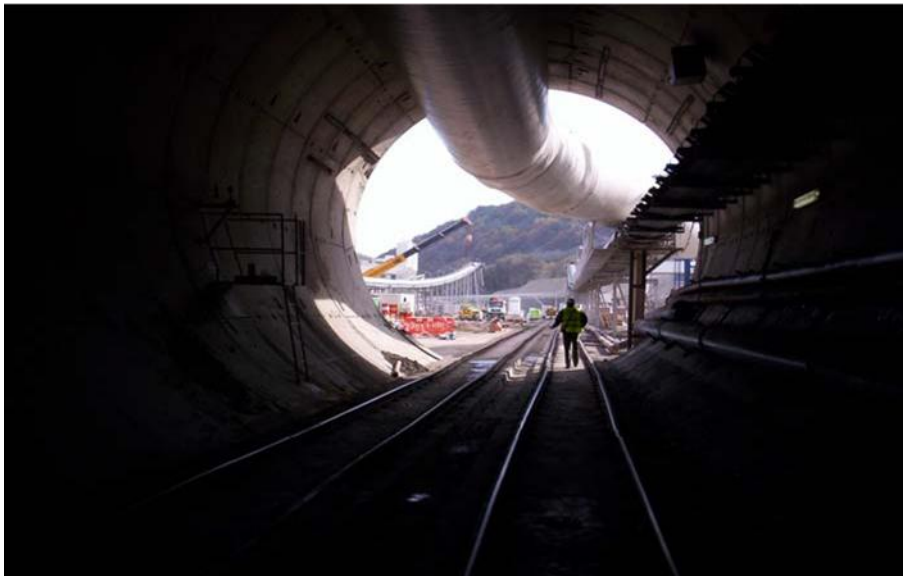
A railway construction tunnel in the North of Spain
